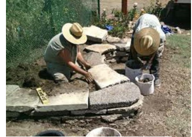
Stone Garden Wall Laying a Broken Concrete
